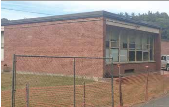
Tech installations will be starting soon on the project.
