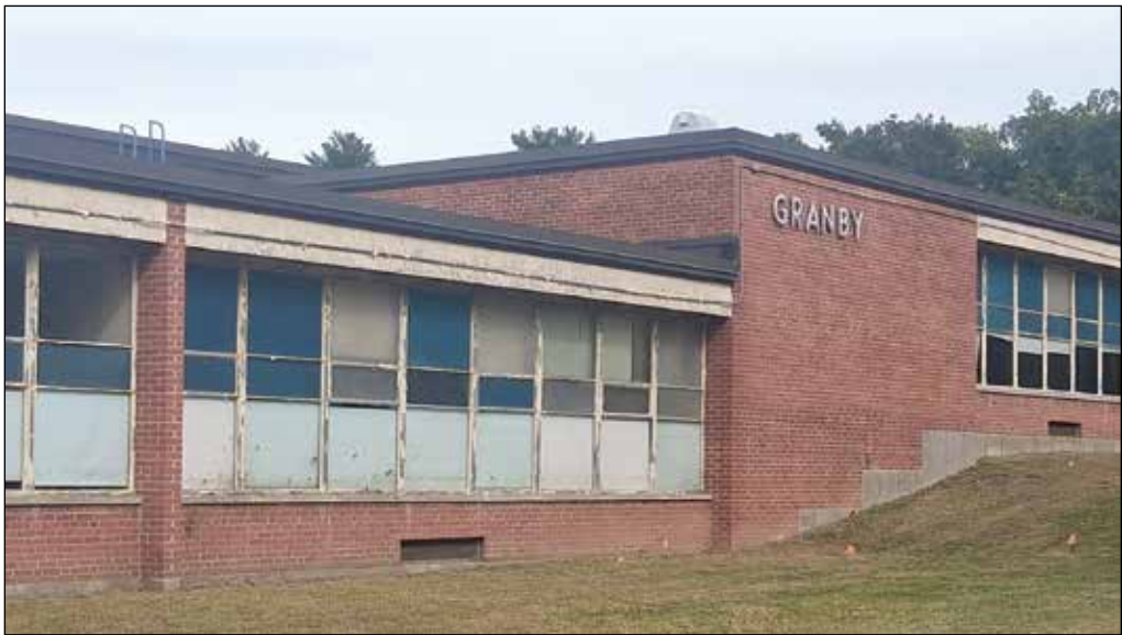
The building is nearing completion of its renovations.
