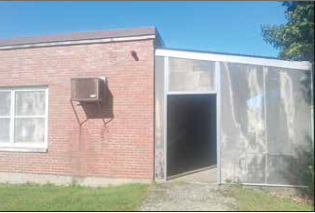
A translucent walkway.
