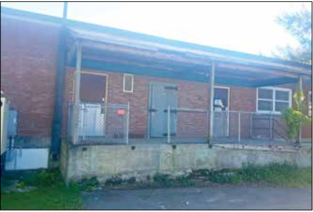
The rear of the building.
