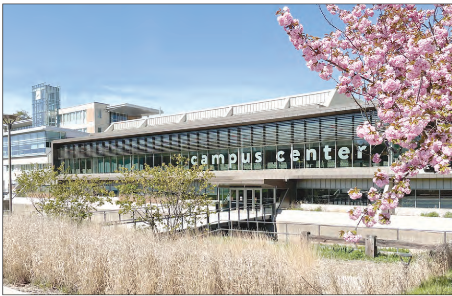
Holyoke Community College's Campus Center
