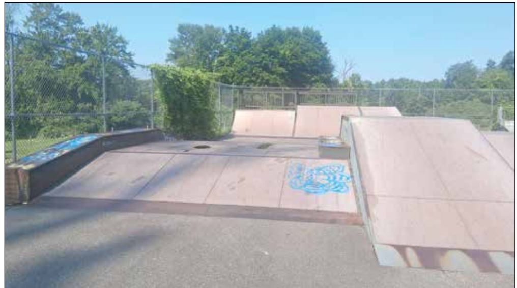
A more detailed shot of the sloped ramps leading to the opposite wall ramps.
