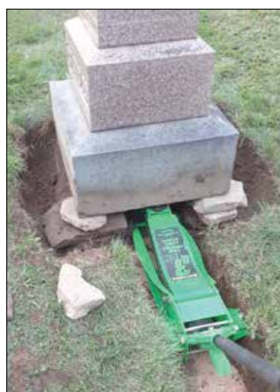
A green leveler lifting up the gravestone so that the ground can be filled in.
