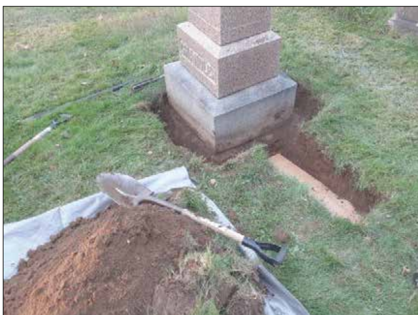
A newly filled hole after the levelling was completed.
