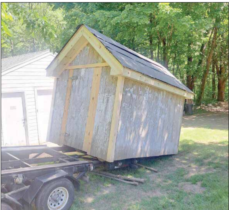
Moving the old shed to its new location, complete with new wood paneling.
